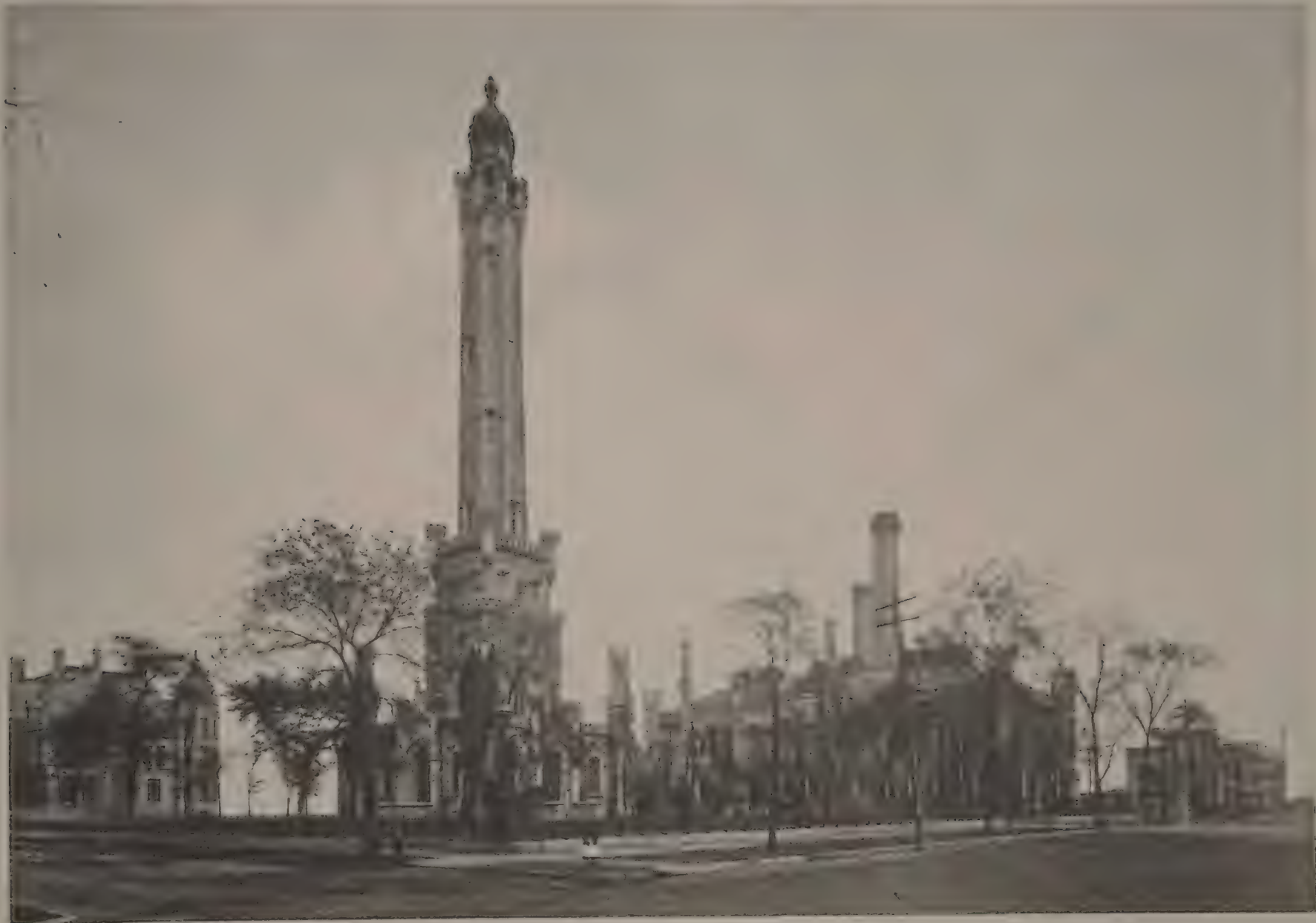
NORTH SIDE WATER WORKS.
